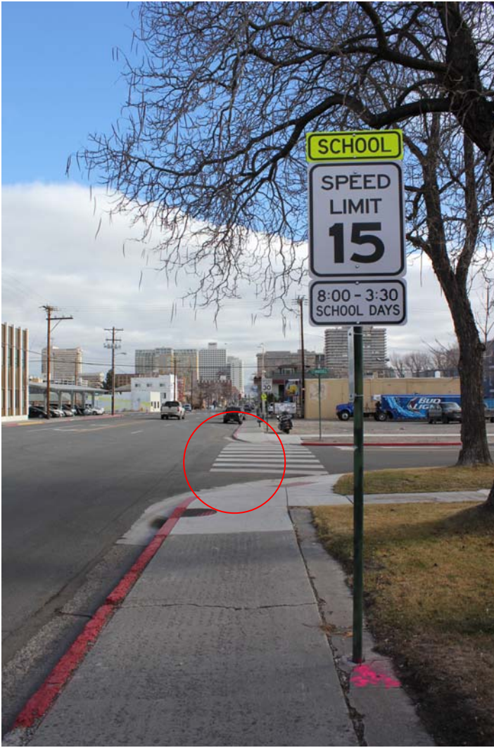
Photo 11 – looking eastbound on 2 nd Street at the intersection of Winter Street showing the new school zone from Winter Street to Washington Street.
