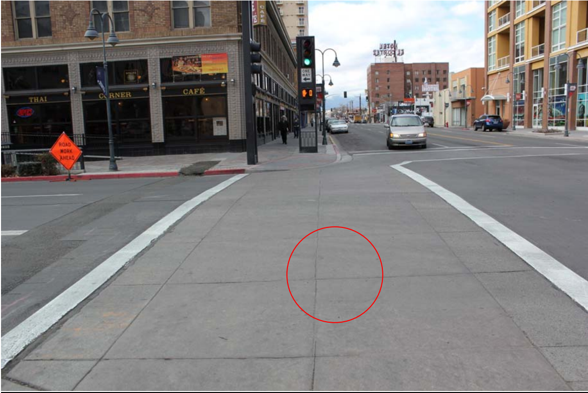
Photo 13 – showing the existing crosswalk on the west leg of the intersection of 2 nd Street and Sierra Street.
