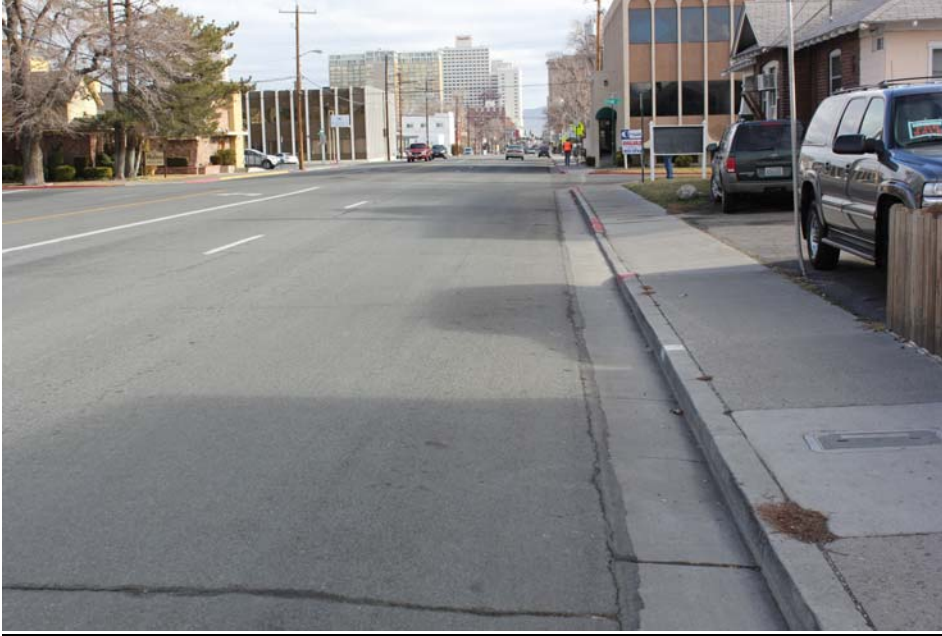
Photo 1 – Typical cross section of the existing roadway on the project
