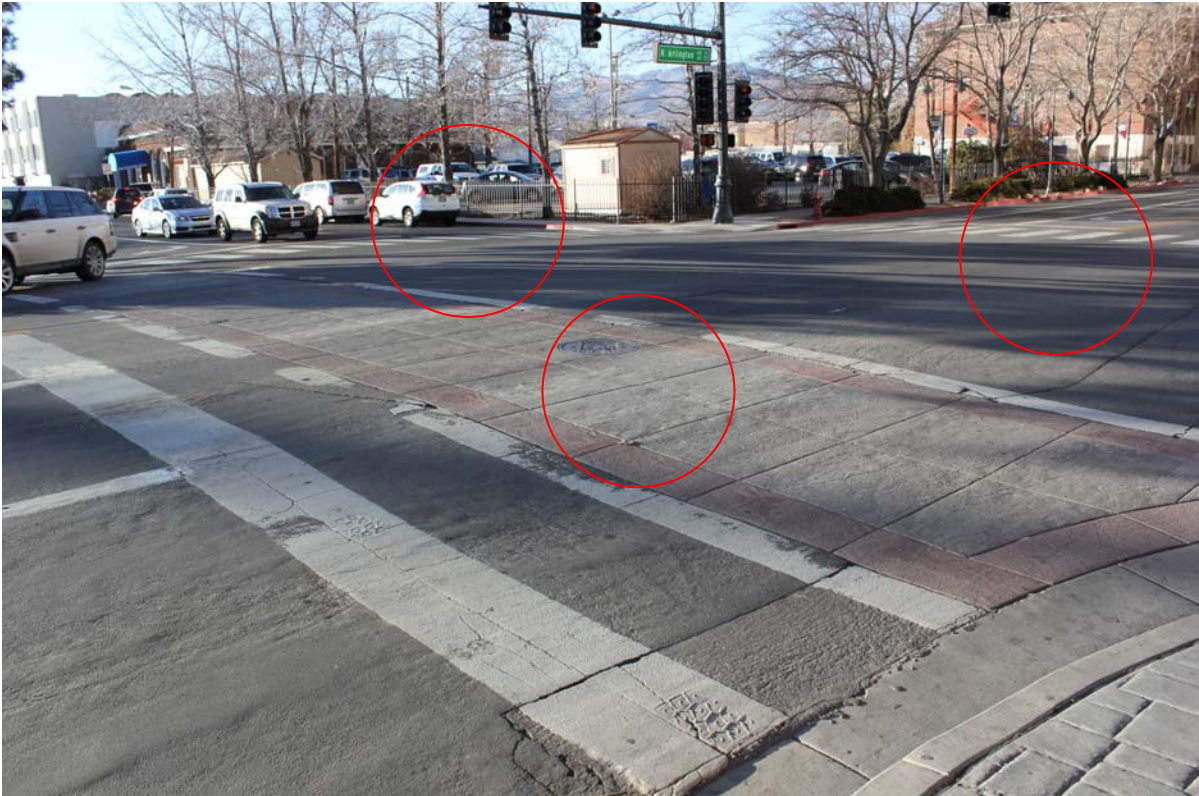
Photo 42 – Looking at the existing crosswalk on the south leg of the intersection of Arlington Avenue and 1 st Street.
