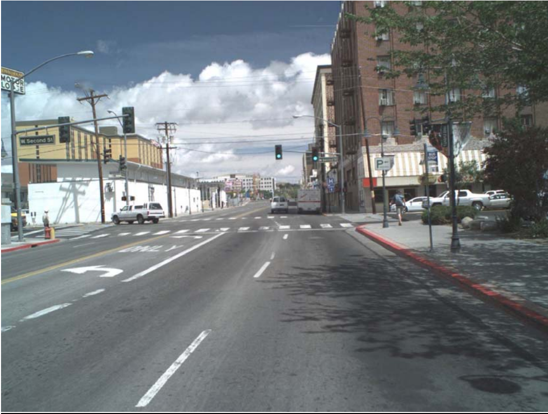
Photo 29 – Typical cross section of the existing roadway on the project
