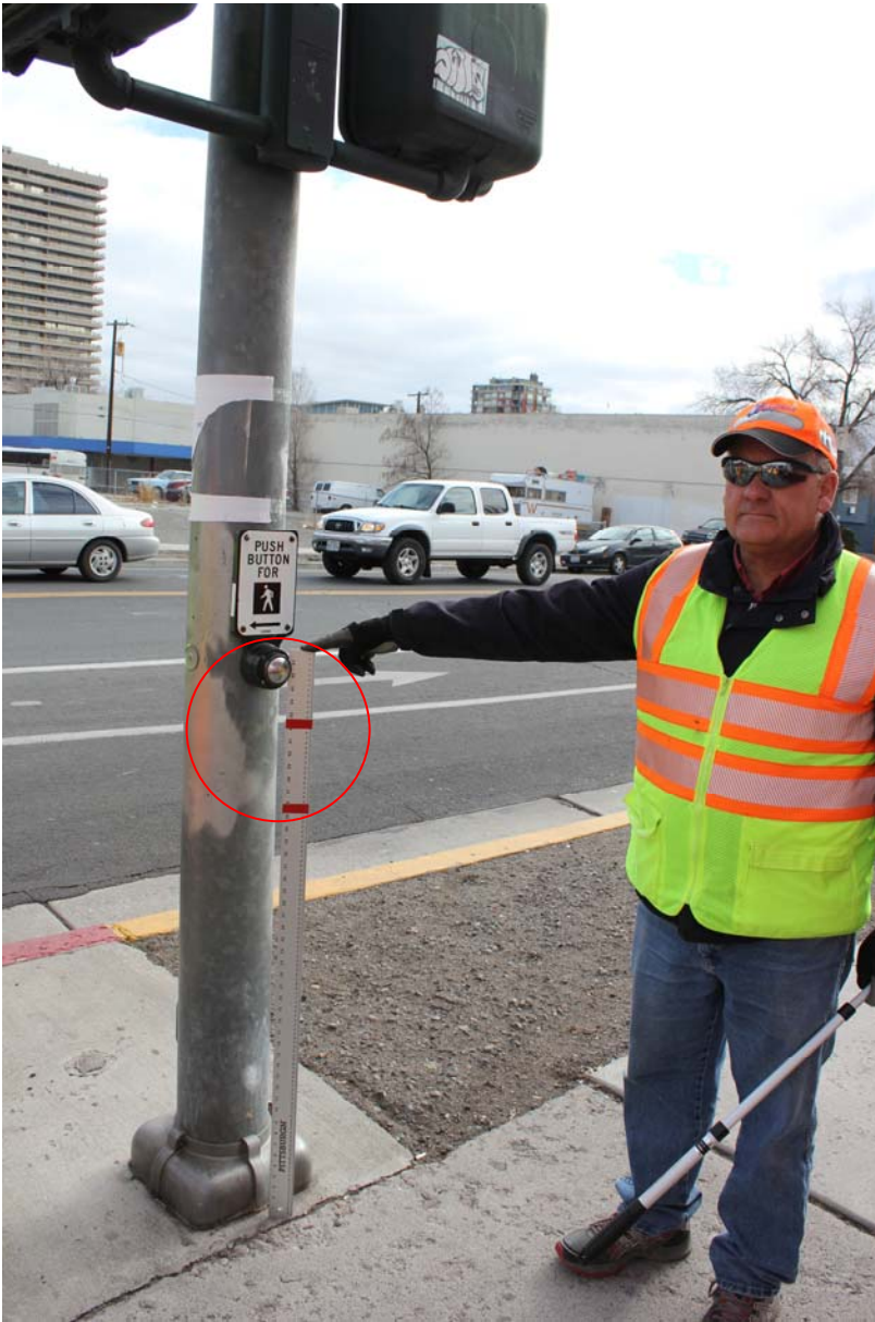
Photo 3 – Pedestrian Push Button is located above the 42 inches maximum height above the sidewalk.
