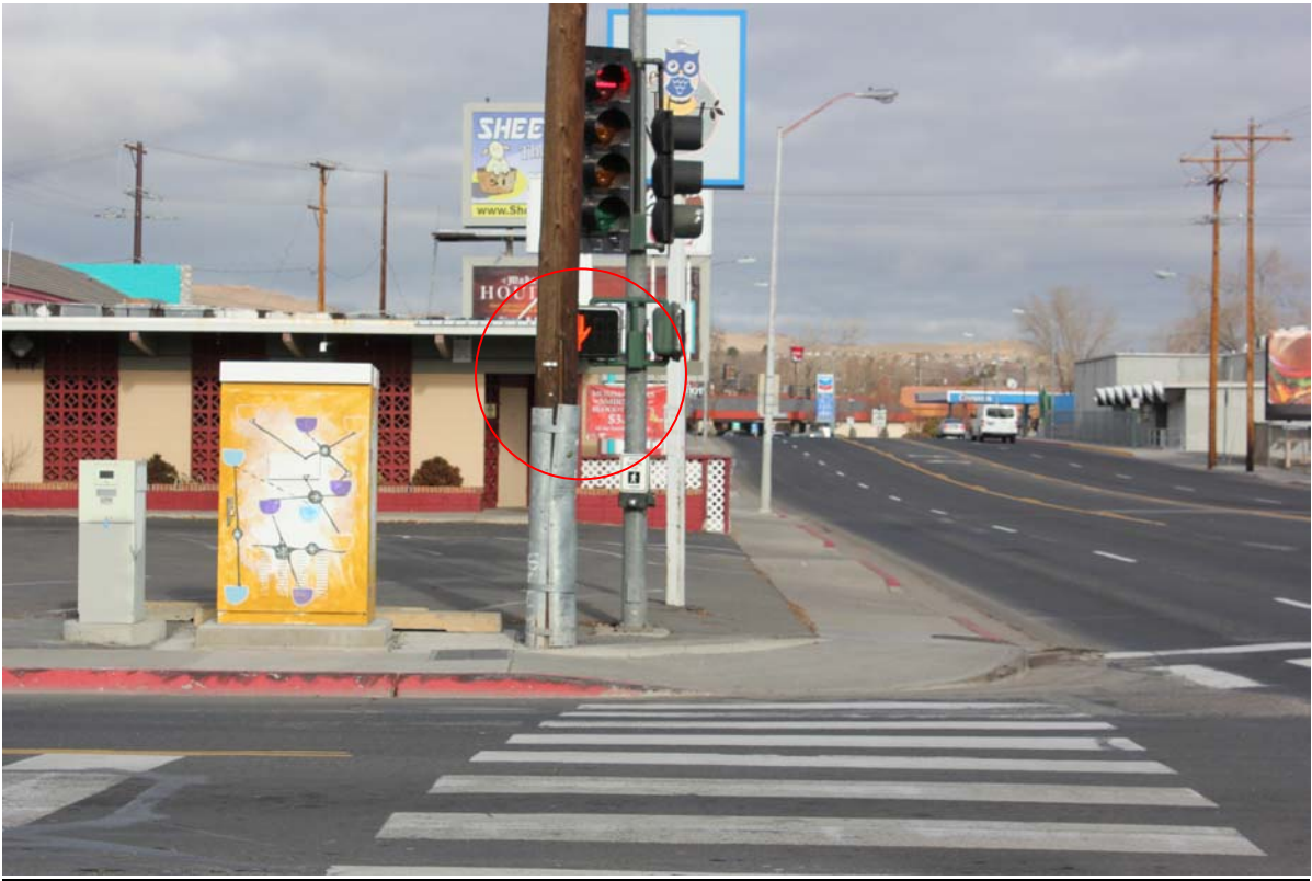
Photo 10 – looking north at the pedestrian signal head on the northwest corner at the intersection of 2 nd Street and Keystone Avenue.
