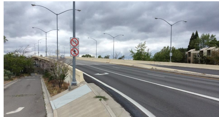
Wells Avenue Bridge over the Truckee River
