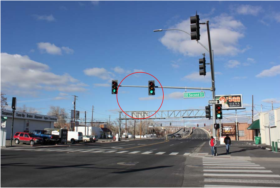
Photo 15 – looking northbound on Wells Avenue at the intersection of 2 nd Street.
