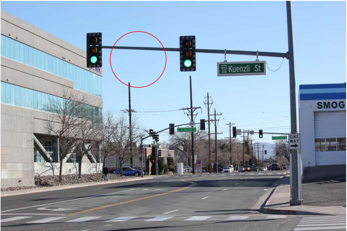
Photo 25 – looking southbound on Kirman Avenue at the intersection of Kuenzli Street.
